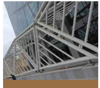
All Types of Steel Structures
