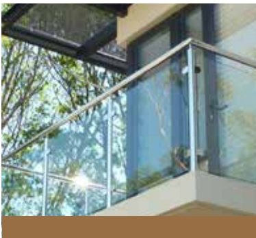
Stainless Steel, Aluminum and Glass Railing.
